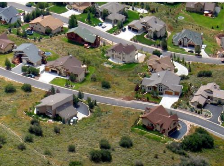
HOME-TO-HOME IGNITION, AS A RESULT OF BURNING EMBERS, CONTRIBUTED TO THE DEVASTATION IN THIS SAN DIEGO, CALIF., NEIGHBORHOOD AS A RESULT OF THE WITCH CREEK WILDFIRE IN OCTOBER 2007.
